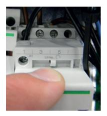
Mount the black wires in the free spaces on the immersion heater.
