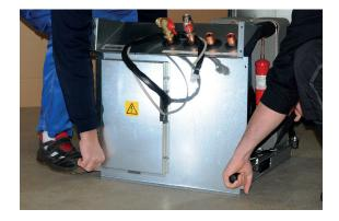
5. Lift the cooling module using the carrying handles and shoulder straps.
