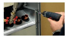
3. Unscrew the cooling module's screws.
