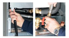
1. Disconnect the cooling module's power cable connector and hoses.
